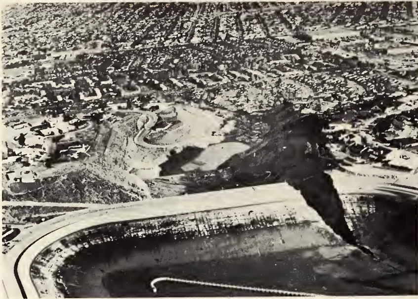
In Los Angeles, Baldwin Hill Reservoir cracked, then broke releasing a torrent which wrecked hundreds of evacuated homes, but produced few casualties.
